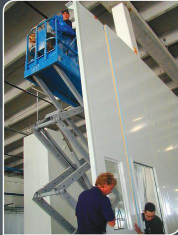
**Panel Replacement:** The non progressive post design provides the ability to swap or replace individual panels without disturbing the adjacent panels.
